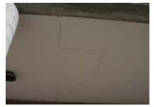
Soffits - Soffits at the Main Gymnasium entrance is warping, bowing and coming loose at the edges and cracking at the seams.
