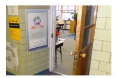
**Pull Side of Doors** - Pull side on entry doors to the classrooms in the main structure are recessed and don't have required 18 inch clearance which does not meet the ADA accessibility code. Modular classrooms have the required clearances.
