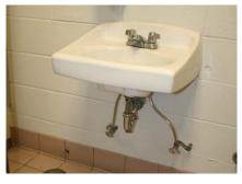
**Lavoratory Sinks-** Some of the ADA accessible sinks do not have the required fixtures or pipe insulation on the pipes below sink.
