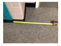
**Pull side Door Clearance** - Pull side of door on multiple classrooms and misc. closets and restrooms throughout the building do not meet the required clearance of 18" clear. Approximately 25 classrooms and 10 miscellaneous spaces do not meet code.
