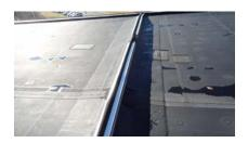
**Roof** - The roof is an EPDM roof system in all areas. There are areas of ponding indicating low areas but overall the roof appears to be in good condition. It has been reported that the most recent repairs were on 705 sqft of the roof and was performed in 2004.
