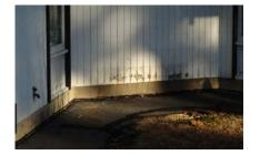
*Exterior Walls* - Exterior walls are painted block and are in fair to good condition. A few areas around structure are in need of attention. Paint chipping or peeling and need repaired at base of panels below down spouts.
