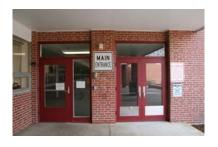
Exterior Walls - Exterior walls of the original 1960 building and all the other additions consist of 4" brick exterior facing and an exterior concrete masonry unit backup. Around the perimeter of the building bricks in the corners are broken, chipped or damaged in a number of areas and require repairing.
