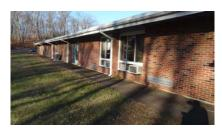
**Exterior Walls** - The exterior walls of the 1957,63 and 88 structure consist of brick masonry with concrete masonry unit backup. The exterior masonry walls appear to be in good condition showing no significant need of remedial work with the exception of some staining and minor cracks. Again, these can be treated, cleaned and patched to provide a more aesthetically pleasing appearance.
