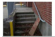
**Loading Dock** - Concrete at loading dock stairs and around platform is cracking, chipping and spalling. Lintel at receiving area entry is rusting. Broken panel below window.
