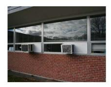
Windows - Existing window units are aluminum framed, single glazed windows and are original. Window AC units also appear to be in poor condition. Painted peeling around wood frame and plywood panel and metal exterior casing is dented or damaged. Glass block windows around Auxiliary Gym are broken and mismatched.
