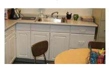
**Sinks** - Sinks in classrooms and workroom do not meet ADA rerequirements. Fixtures on sinks are mounted more than 11 inches from front of counter. Pipes below sinks in do not have pipe insulation.
