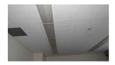
**Ceilings** - Most spaces have 1x1 ceiling tiles installed and were noted to be in fair to poor condition (See Hazardous Material section). Suspended acoustical ceilings were installed in the modular classrooms and were noted to be in fair to good condition on average.
