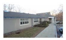
*Exterior Walls* - Exterior walls of the original building was refinished in 1997 applying the stucco exterior facing. Exterior appears to be in good condition.
