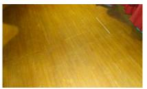
**Flooring** -Majority of the flooring is carpet and is located throughout the building. These are in fair to good condition. Platform or Stage flooring is a stained wood and is in need of refinishing. A few areas have VCT flooring and are noted in the Hazardous section.
