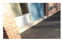
*Exterior Doors* - Multiple exterior doors, around entire building, exit to a step down area and not a platform or ramp.
