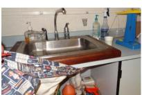
*Sink Fixtures* - Fixtures on the sinks in the classrooms are not ADA code compliant. Fixtures are required to be no more than 11 inches from the front edge of counter.
