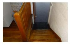
**Stage or Platform Stairs** - Platform which shares space with the Cafeteria has 4 risers up to the stage. There are no extensions at the top or bottom of stairs as required per current codes.
