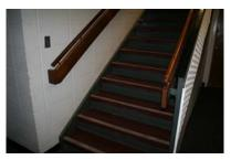
*Stairs* - Stairs do not have the required handrails and extensions at top or bottom.
