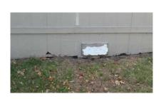
**Portable Classroom Modular**- The painted wood paneling and trim are in good condition but the wood skirt around modular's is rotting and or stained in multiple areas at grade level. Stairs and ramps to portable classrooms are in good condition but the stairs need a few code upgrades. (See ADA/ Accessibility Section)
