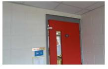
*Interior Walls* - The interior corridor walls and classroom partitions are mainly painted concrete masonry units and in fair to good condition.
