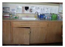
*Sinks* - Fixtures at the sinks in the Faculty Room, Science Room and Nurses office are not ADA compliant. Fixtures on sinks are mounted more than 11 inches from front of counter and fixtures need to be lever or auto flow type.
