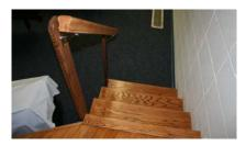
*Stage or Platform Stairs* - Platform has 4 risers up to the stage. There are no code compliant handrails or extensions at the top or bottom of stairs as required per current codes.
