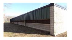
*Windows* - Existing units are metal single pane units and were installed in 1970 and 71 and are in fair condition.
