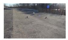
**Roof** - The roof is a modified built-up tar and gravel asphalt roofing system in all areas with the exception of the Portable or Modular units which is a EPDM roof system. There are areas of ponding indicating low areas between the 1957 original structure and the 1963 addition. It has been reported that the most recent roofing work on the Main building was performed on May 1st, 1982. Leaks have been reported in these areas but overall the roof appears to be in fair condition.
