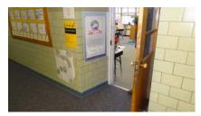
**Doors and Frames** - Solid core wood doors are mounted in hollow metal door frames throughout the building. Many doors have shown signs of wear and should be repainted but are in fair condition.
