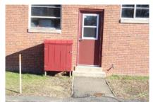
*Exterior Doors* - Multiple exterior doors exit to a step down area and not a platform or ramp.
