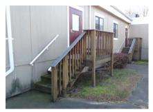
Exterior Stairs - Do not meet current ADA requirements. Rear Entry stair from modular classrooms do not have code compliant hand or guardrails with extensions top or bottom and stairs from Gymnasium do
