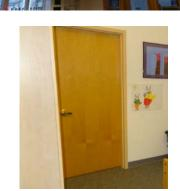
**Doors and Frames** - Solid core wood doors are mounted in hollow metal door frames throughout the building. Doors appear to be in good condition.
