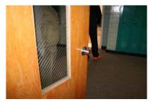
**Knobs on Doors** - Some of the doors on the interior and exterior have knob type hardware which require lever type.
