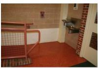
**Ramps** - 2 Ramps at the entrance near the Media Center have drinking fountains at the bottom. Handrail extensions appear to extend into the 5 foot clearance area of the drinking fountains. Recommend wrapping the handrail around the guardrail instead of extending out the 12".
