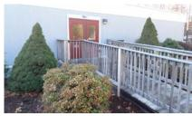
*Exterior Ramp* - Exit ramp from portable classrooms is non ADA compliant. The handrails do not extend at top or bottom of ramp.
