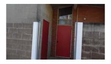
**Doors and Frames** - Exterior hollow metal doors and frames are original to the year the structures were built and doors and frames are showing signs of wear from age and are fading and hardware does not meet the current codes. (see ADA/ Accessibility section) They appear to be in fair to poor condition.
