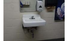
*Pipe Insulation* - pipe insulation miss below ADA sinks in restrooms and classrooms.
