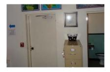
**Panic Hardware:** Exterior door from Special Needs, Room 1A has a knob on door and is required by code to have push bar or panic hardware.
