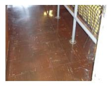
**Flooring** - Majority of the flooring is vinyl asbestos tile and is located throughout the building. (See Hazardous Section) Carpet has been installed in some of the classrooms, kitchen and Hallways over existing tile. These are in fair to poor condition. Platform or Stage flooring is a stained wood and is in good condition but stage is used as an office.
