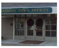
**Doors and Frames** - Exterior doors were replaced in 1997 and are in good condition.
