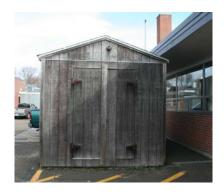
Exterior Wood Sheds - Shed structure near Greenhouse, Tennis courts and outside of Science rooms 40 and 41 are in poor condition. Plywood is flaking and rotting. Paint is fading and chipping.
