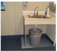
Sink Fixtures - Fixtures on the sinks in the classrooms are not ADA code compliant. Fixtures are required to be no more than 11 inches from the front edge of counter.
