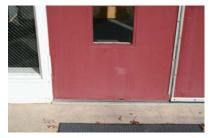
Doors and Frames - Exterior doors appear original to building and are in fair to poor condition. Doors and frames are either fading, oxidizing or rusting and missing either weather stripping or bug sweeps.
