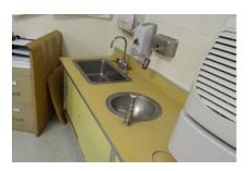
**Laminated Casework** - The laminate on the casework in almost all classrooms and offices are old and showing signs of age and are chipping or peeling.
