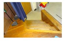
Stage or Platform Stairs - Platform which shares space with the Gym/Cafeteria does not have ADA accessibility. No ramp stairs that have 5 risers up to the stage. There are no handrails with extensions at the top or bottom of stairs as required per current codes.
